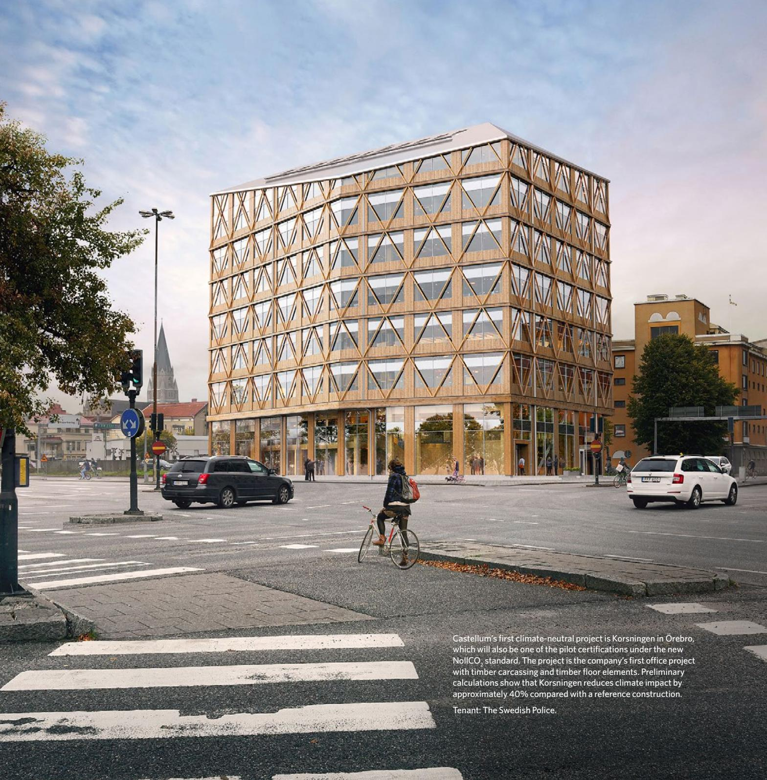
Castellum's first climate-neutral project is Korsningen in Örebro, which will also be one of the pilot certifications under the new NollCO<sub>2</sub> standard. The project is the company's first office project with timber carcassing and timber floor elements. Preliminary calculations show that Korsningen reduces climate impact by approximately 40% compared with a reference construction. Tenant: The Swedish Police.
